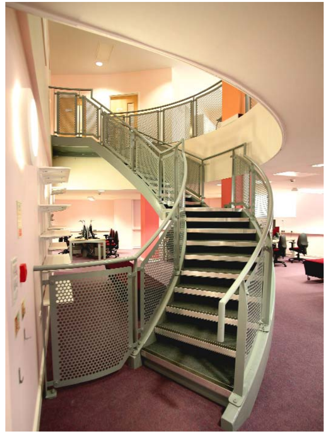
Half spiral staircase links the two floors
